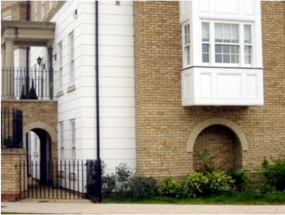
Fig 8: external nook at Beaulieu Park (on The Aragon house)
