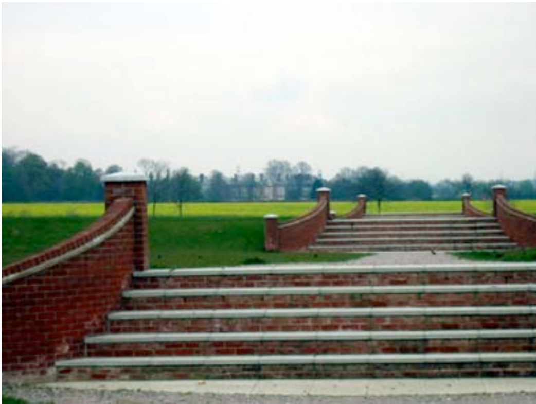
Fig 15: view through to New Hall today
